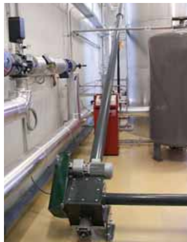
For example, this ascending worm screw carries the falling ash from 2 HERZ systems over a height of approximately 4m, to a 2m³ sized ash container which is placed outside the heating facilities.
