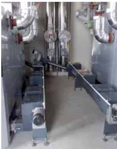
This image shows the ash container of a 2 HERZ boiler cascade solution connected via the screw system.
